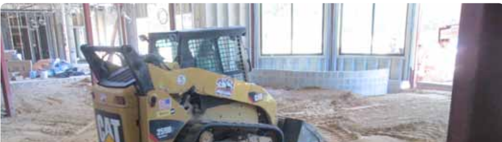
A 6-foot Mashpee Wampanoag Tribal logo will be uniquely designed as part of the Terrazzo flooring as well for all of the Tribal members and visitors to see as they walk through the doors.
